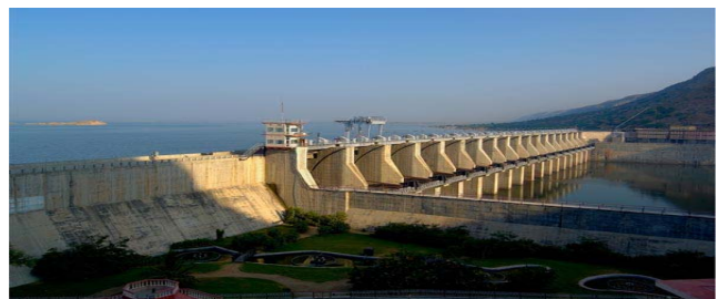
Fig. 1 Bisalpur Dam Site
